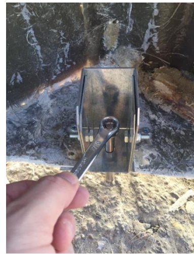
Place anchor and tighten
